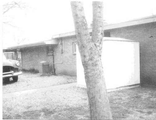
REAR VIEW OF SUBJECT
